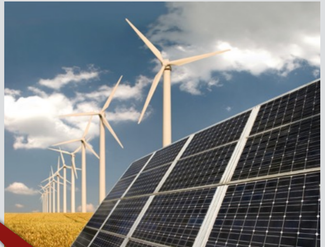
Power generation networks
