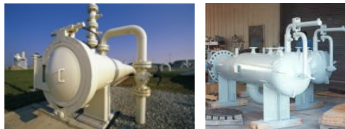
Fig. B.8 Pig Launcher, Receiver
