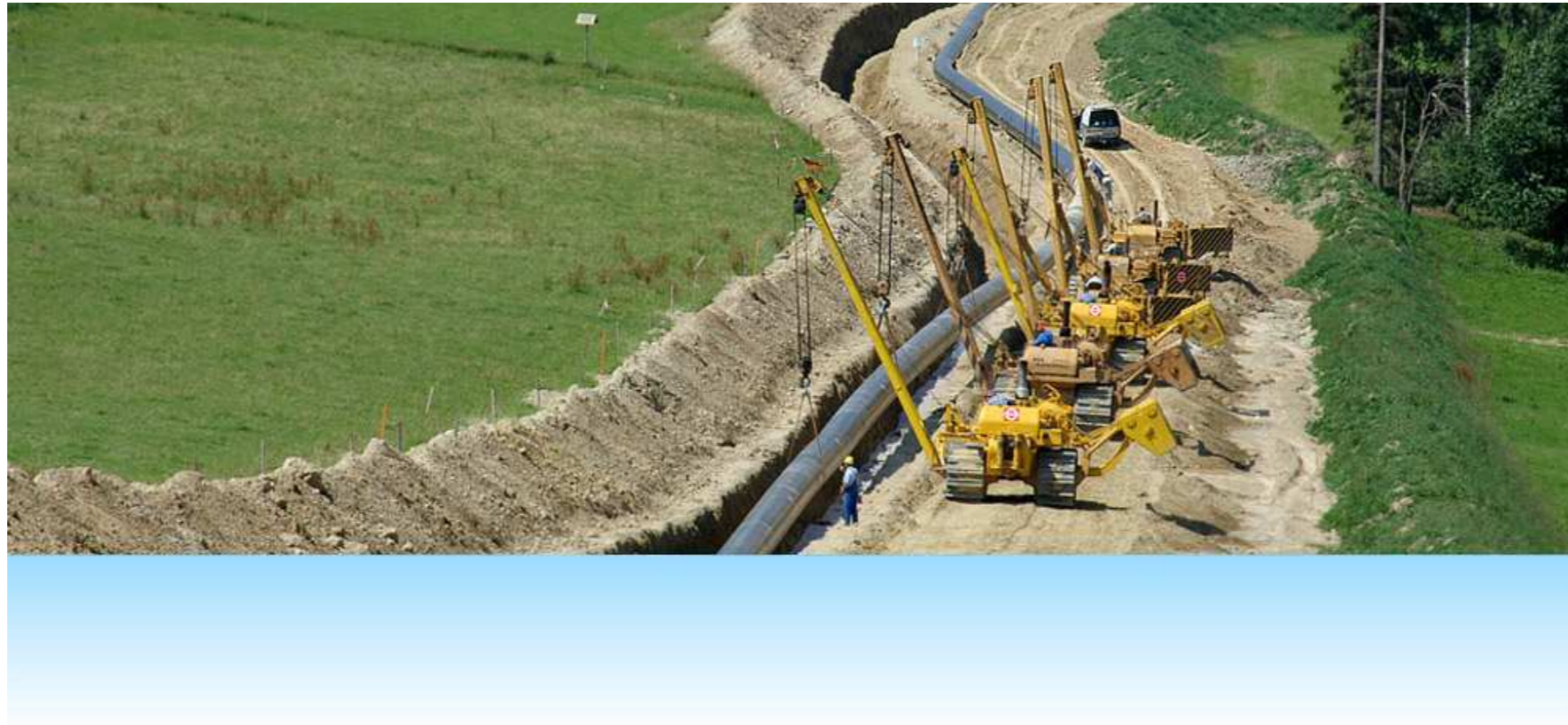
Figure B.4: Pipeline Construction
