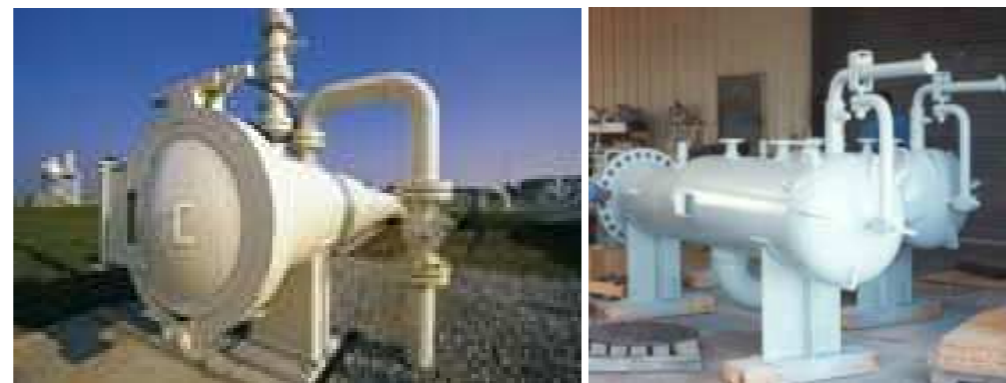
Figure B.10: Pig Launcher, Receiver
