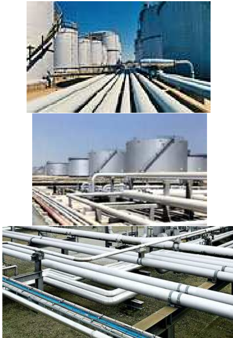
Fig. 5.7 Oil and Gas Switches
