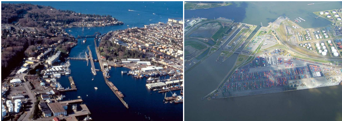
Fig. 0.17 Harbour Canal Locks
