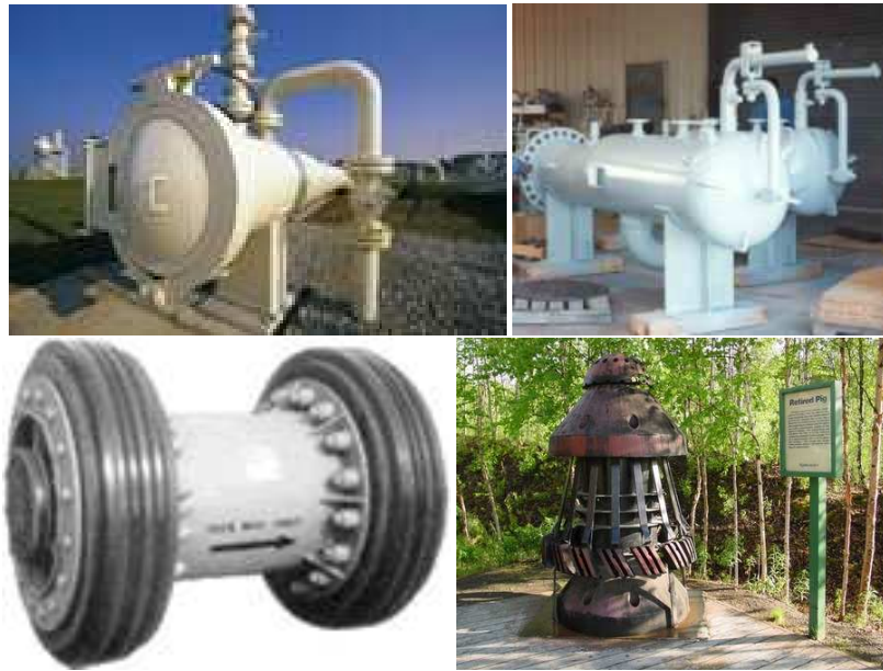
Fig. 5.9 To be treated in a later version of this report: Pig Launcher, Receiver and New and Old Pigs
