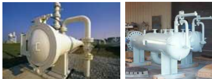
Fig. B.8 Pig Launcher, Receiver
