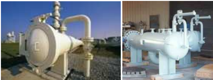
Fig. B.10 Pig Launcher, Receiver
