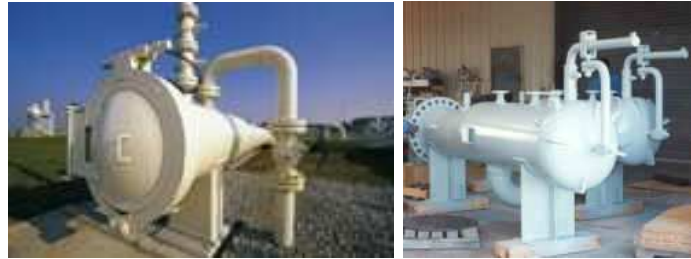
Figure 10: Pig Launcher, Receiver
