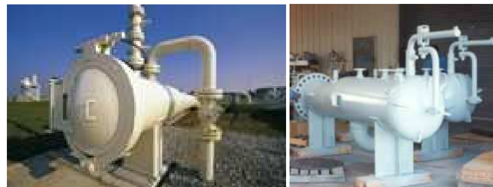
Figure B.9: Pig Launcher, Receiver
