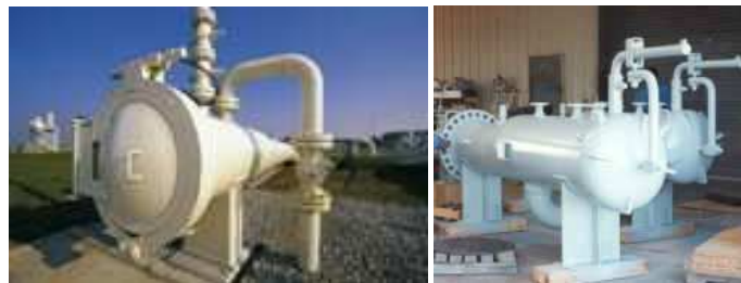
Fig. B.9 Pig Launcher, Receiver
