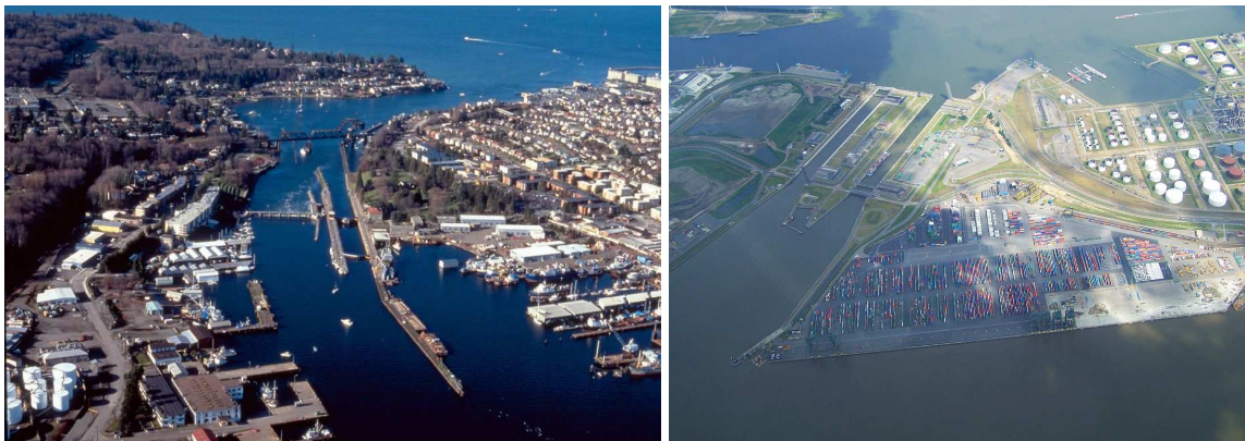
Figure 9: Harbour Canal Locks
