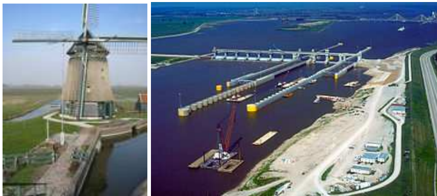
Figure 37: Polder Pump (NL) and River Lock (US)
