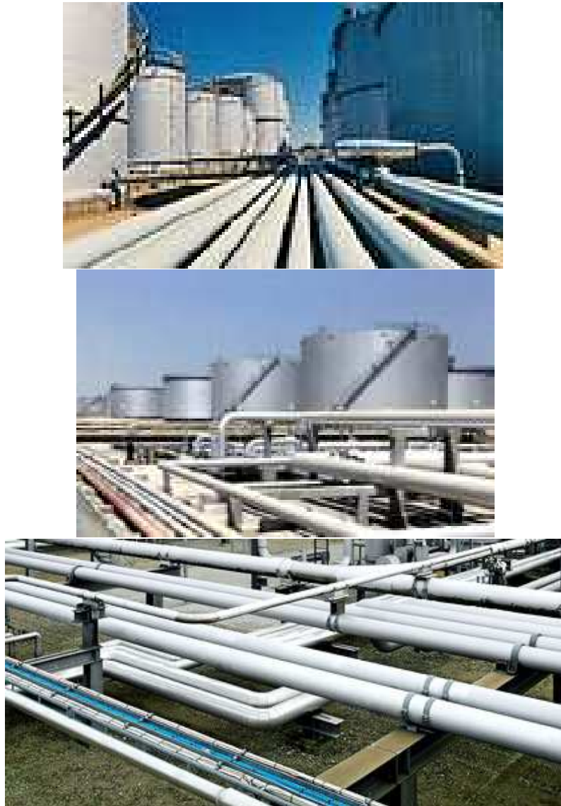
Fig. C.7. Oil and Gas Switches
