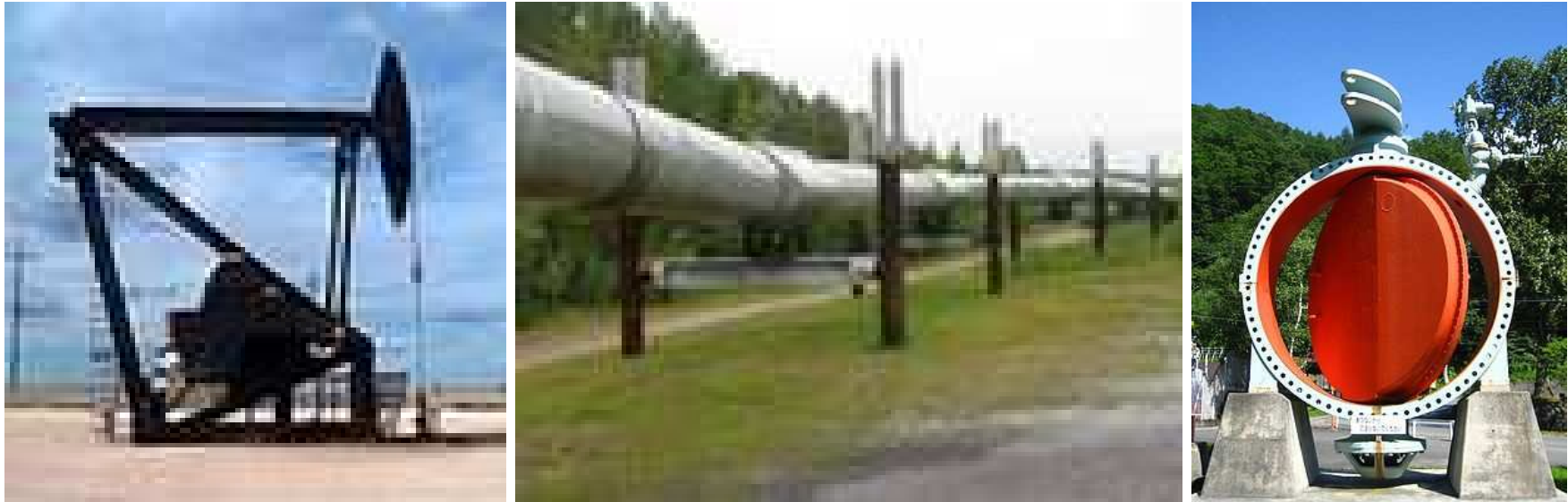
Figure 2: Pump, pipe and valve pipeline units
