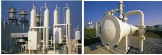
Fig. F.10. Gas Cleansing: Glycon Drying Station and Gas Pig
